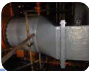
Cold water lines operating in a high humidity environment coated with 361 Thermal Barrier
